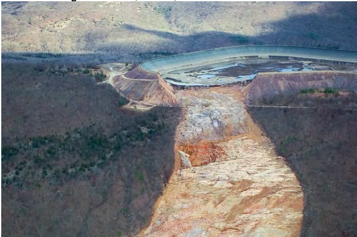
Taum Sauk Ring Dam Failure, Dec. 14, 2005
