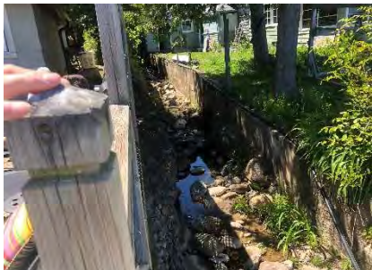
Typical Cedar Ave Storm Drain, May 2026
