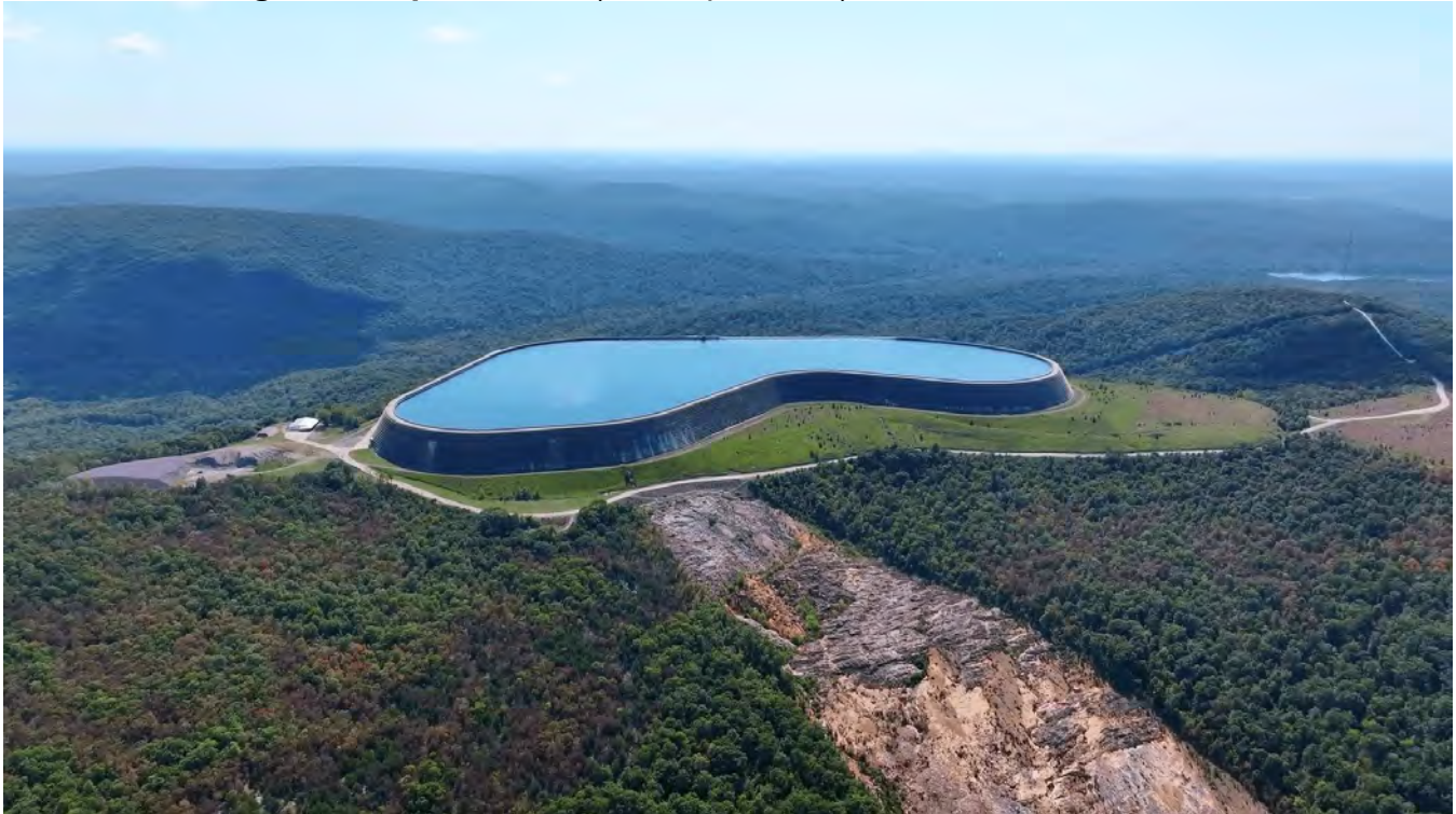
Taum Sauk Ring Dam Replacement (circa April 2010)
