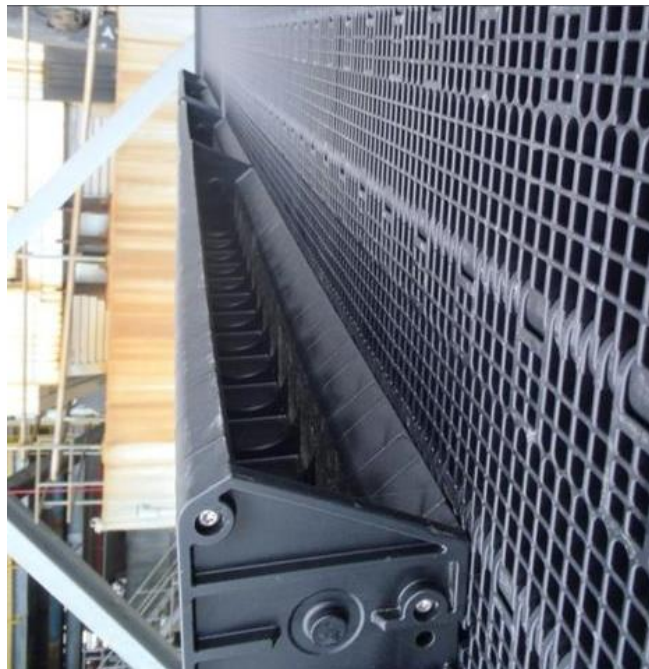
Figure 4-9 Hydrolox Screen Mesh and Fish Bucket (Courtesy of Alden).
