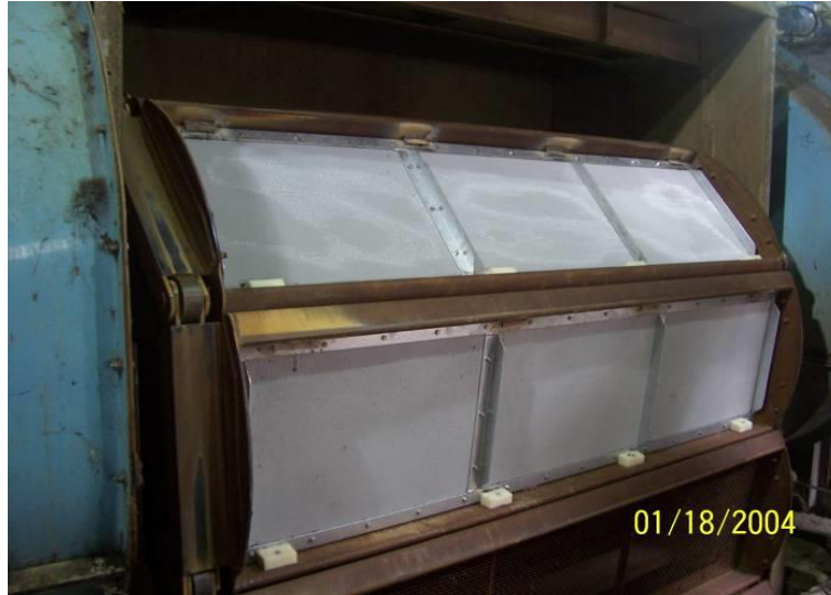
Figure 4-7 Traveling Water Screen with Fine-mesh Overlays (Courtesy of Alden)
