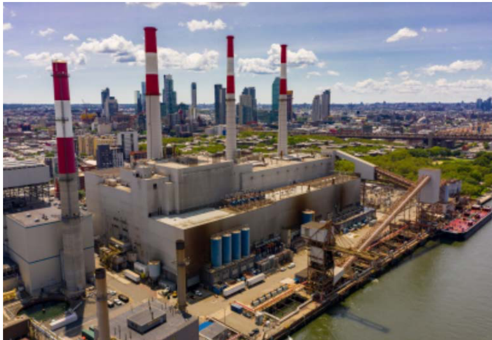
Figure 6-5: New York Approves 316 MW Battery Plant
