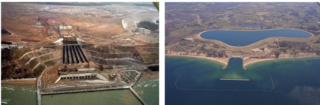
Ludington during construction (left) and operational (right)
