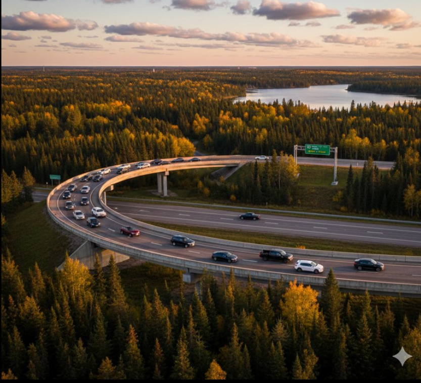
Highway 17 overpass near Ignace to allow NWMO employees on their daily commute to the Revell DGR site, to cross to the north side, where the feeder merges with the west-bound side.
