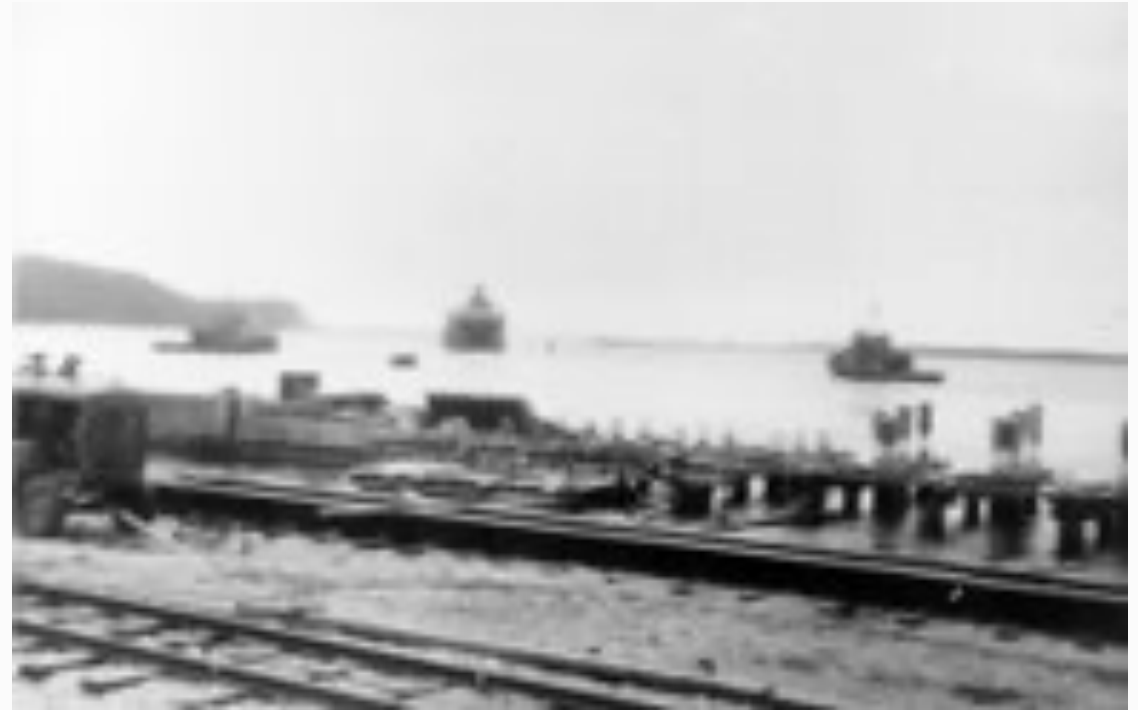
Port of Stephenville under construction 1951
