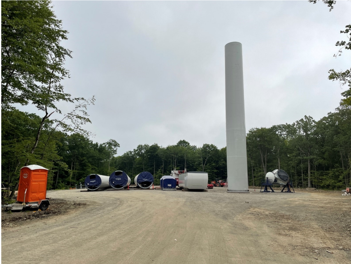
Lay down area
