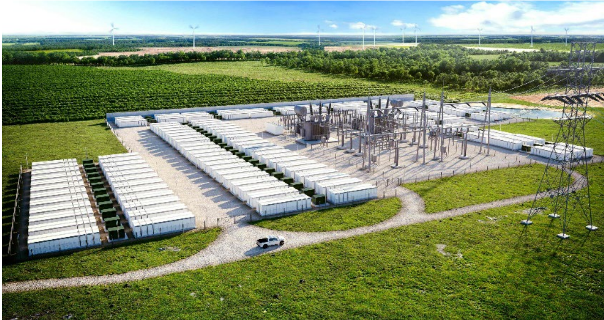
Rendering of NRStor and Six Nations of the Grand River Development Corporation's 250MW / 1000MWh Lithium Ion Oneida Energy Storage Project located in Ontario, currently under construction.
