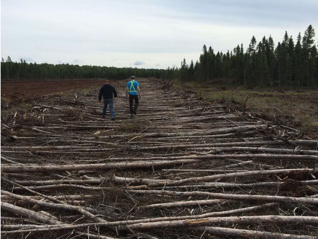
Photo 4.3-1: Corduroy road during its construction, before adding the layer of clay.
