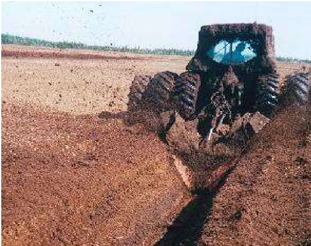
Photo 4.2-1: Picture showing a V-ditcher digging a secondary ditch
