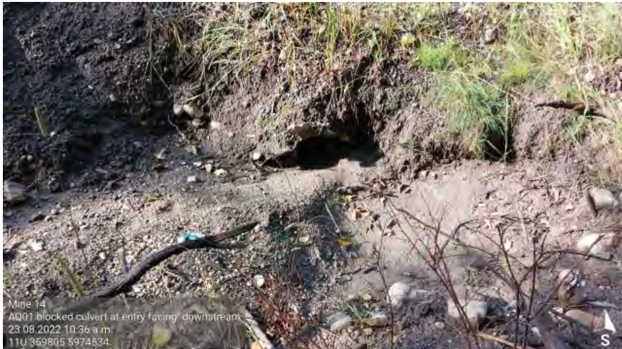
Picture 5: Blocked culvert under existing road.
