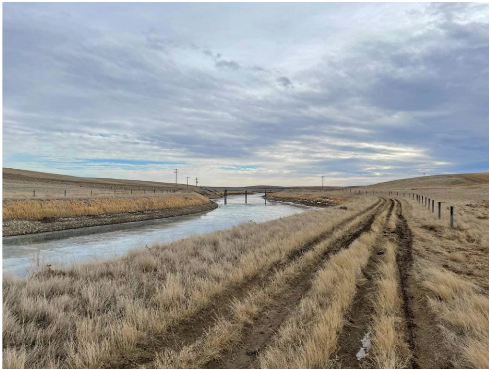
Photo 1: Main Dam Looking Downstream on Main Canal January 2022
