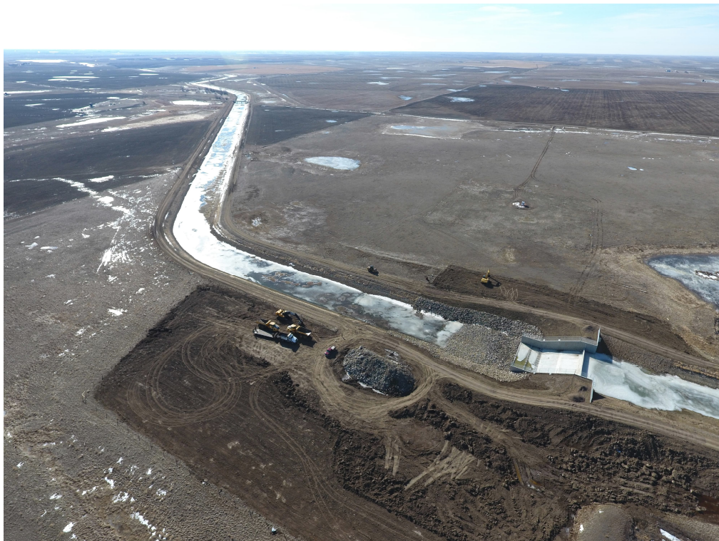
Photo 4: Reservoir Inlet Structure and Future Reservoir Area, March 2019
