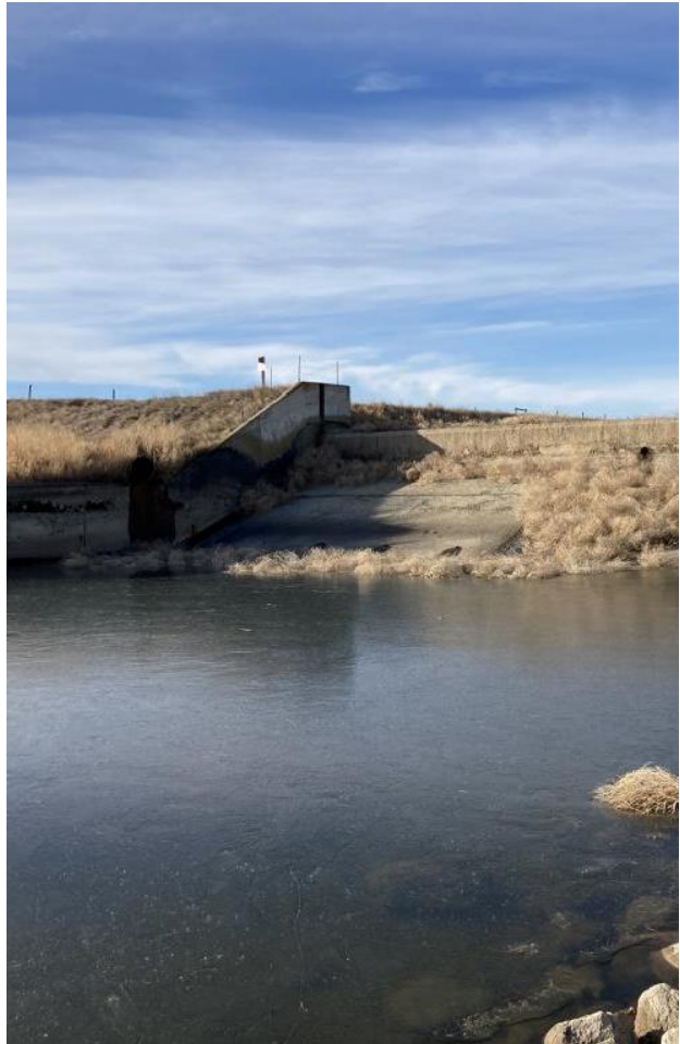
Plate 16. Pooling downstream of weir at Area 4
