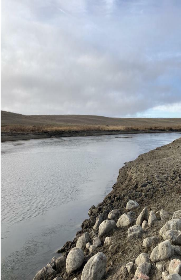
Plate 17. Upstream at Area 5
