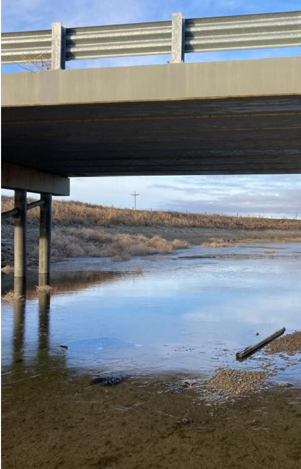
Plate 1. Upstream at Area 1
