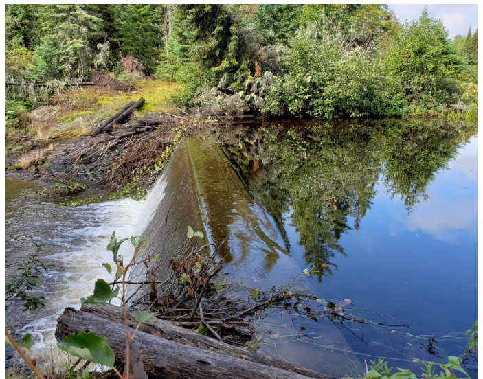
Hydrology station on Victoria Creek, upstream of the Upper Beaver Project area.
