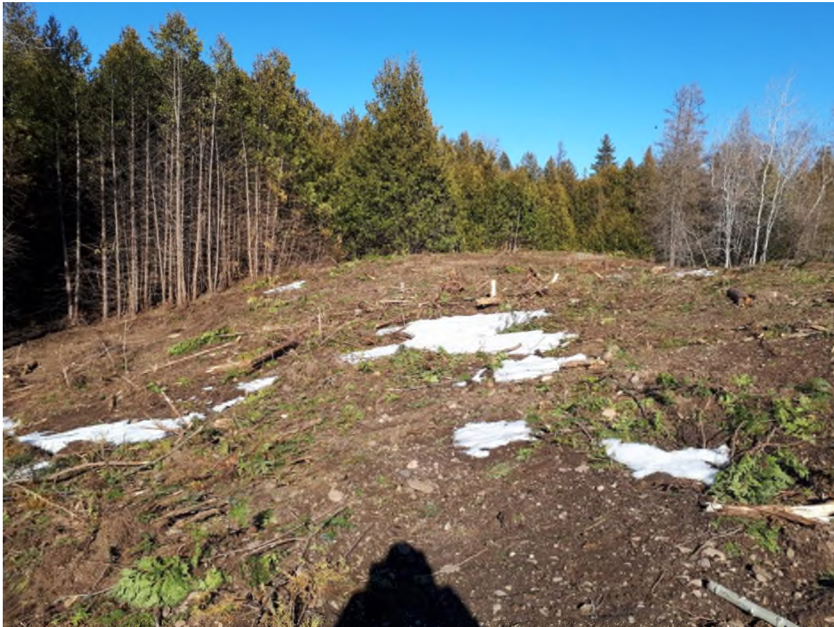
Photo 5. Looking East Tree Clearing
